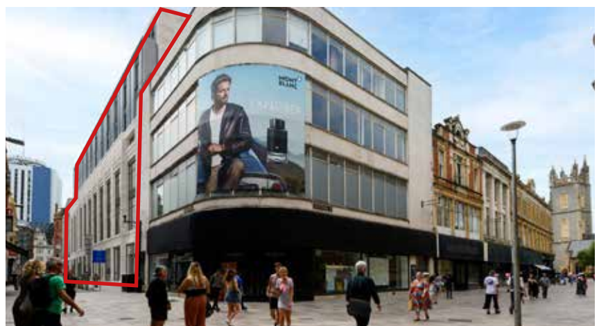
Former Howell's Department Store, Patel Taylor Architects
