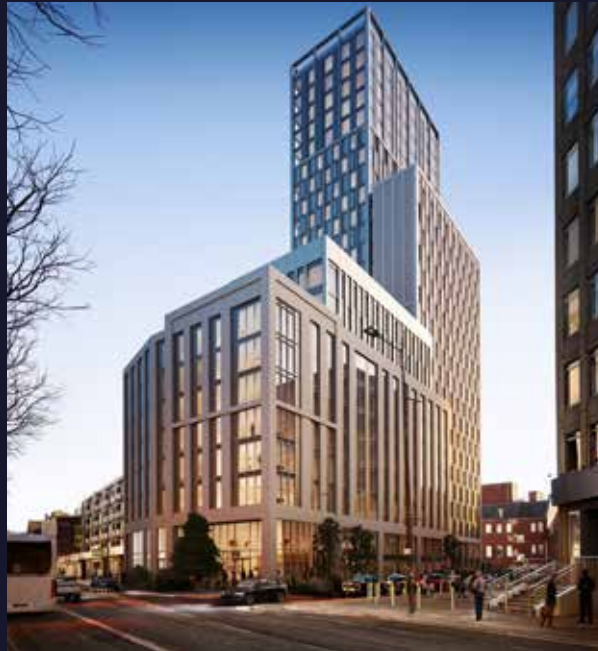
Friary House, Greyfriar's Road Westworks Architects and Rio Architects
